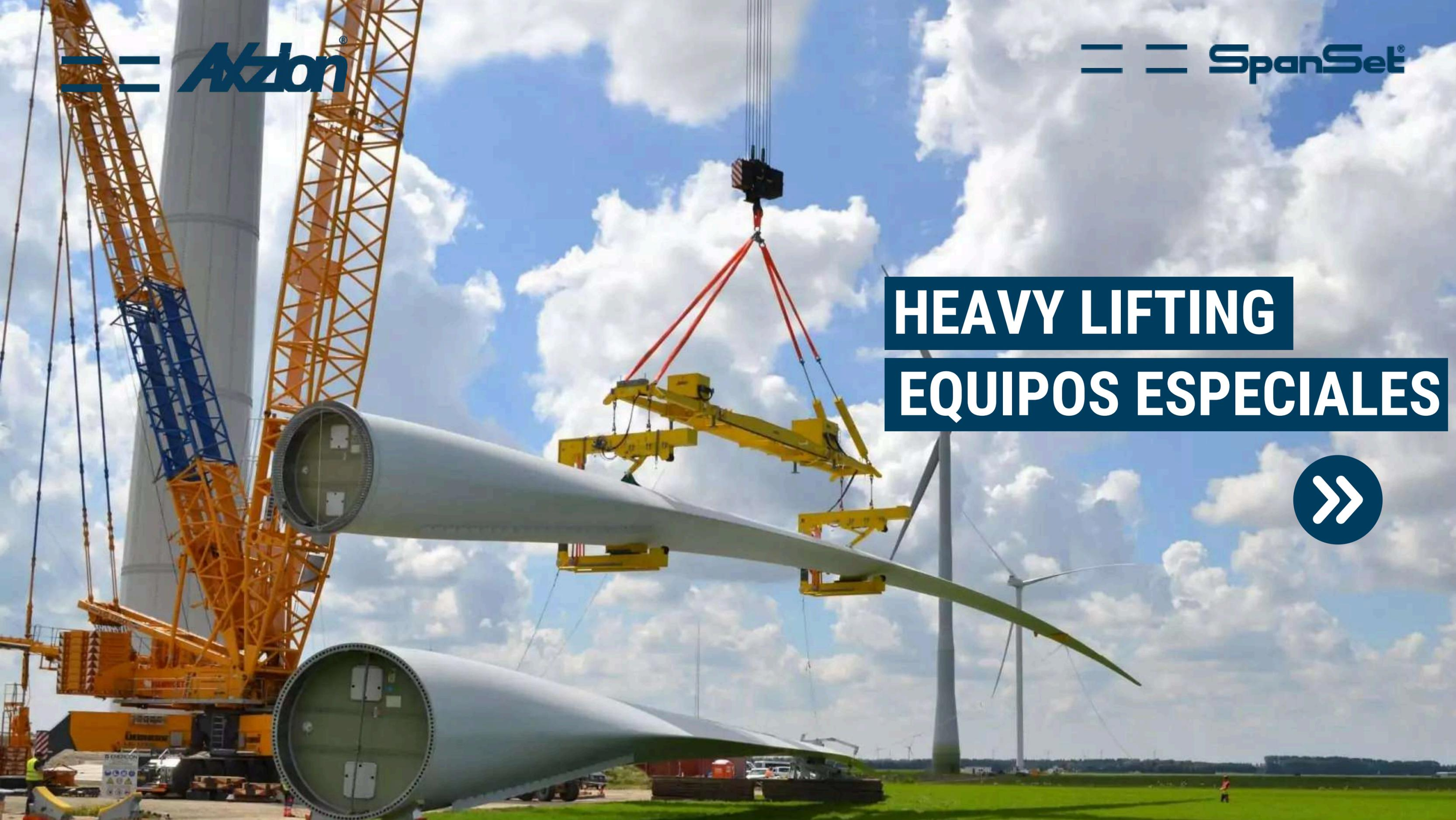
A large white wind turbine blade is being lifted by a yellow crane using a yellow SpanSet lifting beam and red slings. The scene is set outdoors on a grassy field under a blue sky with white clouds. Other wind turbine towers and blades are visible in the background.
