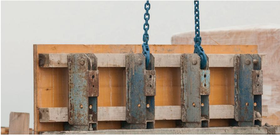
**2-Leg Chain Sling with Shortener and Clevis Sling Hook EXOSET®**
