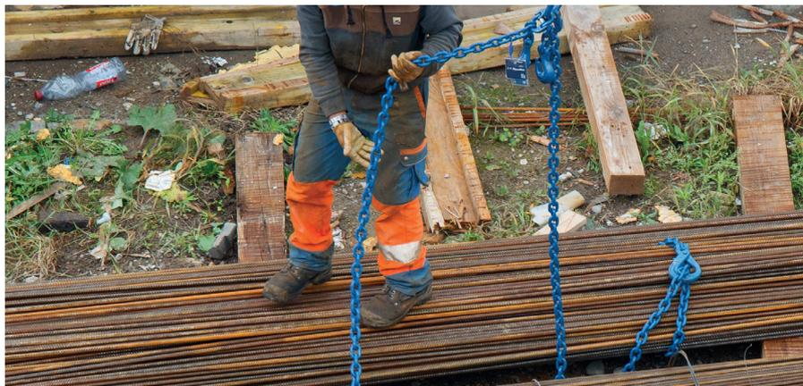
**4-Leg Chain Sling with Shortener and Clevis Sling Hook EXOSET®**
