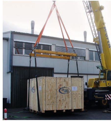
Spreader beam suspension connection below the centre of load point
